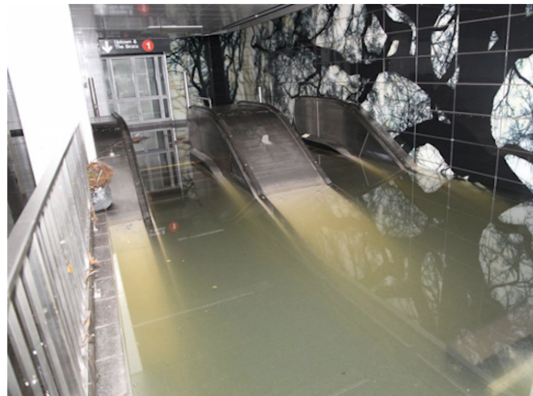
South Ferry Subway (Oct. 2012)
